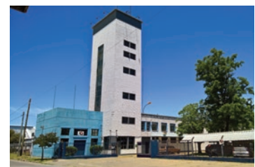
Manufacturing Facility Buenos Aires, Argentina
